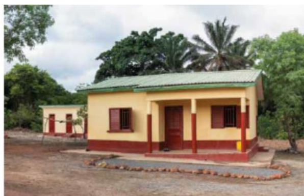
Figure 13. Modern houses equipped with electricity for displaced households [6].
